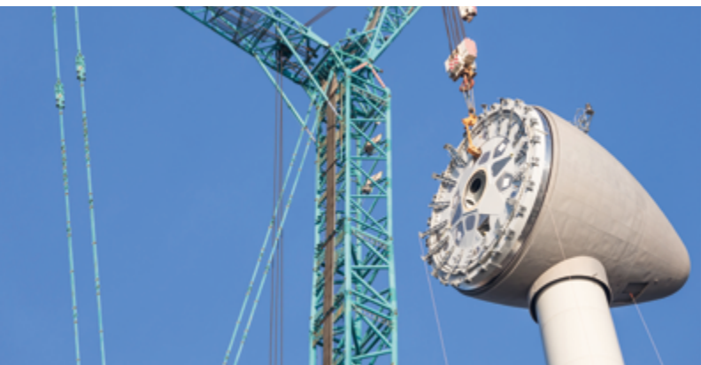
Turbine installation and assembly
